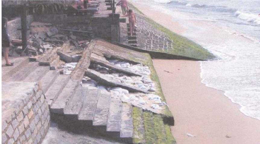
**Fig. 10:** Seawalls destroyed by erosion processes at the limit of the western resorts
